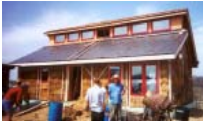
Fig 13: Test house with Bales installed, ready for earth and lime plaster
