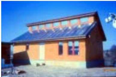
Fig 14: Test house with earth and lime plaster and roof solar hot air system installed
