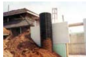
Fig 11: Earth tube system installation, test house
