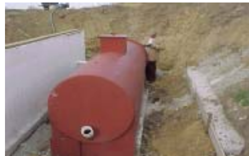
Fig. 8: Methane Digester Installation
